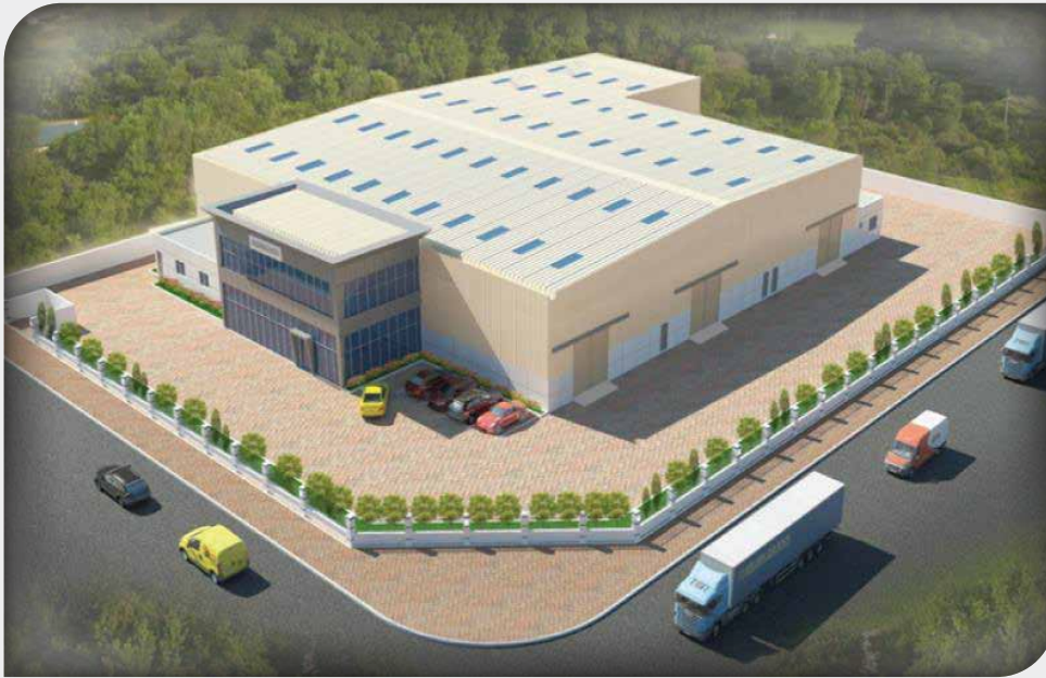
Warehouse & Office at DIC P.N-5330257 Sub-contractor
